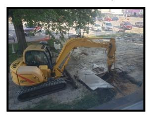
Courthouse sidewalks were removed in order to install piping for the new geothermal heating and cooling system.
